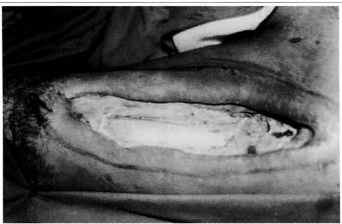
Fig. 1 – Area of radio necrosis on the front side of the thigh. Debridement area marked with an adequate margin.
